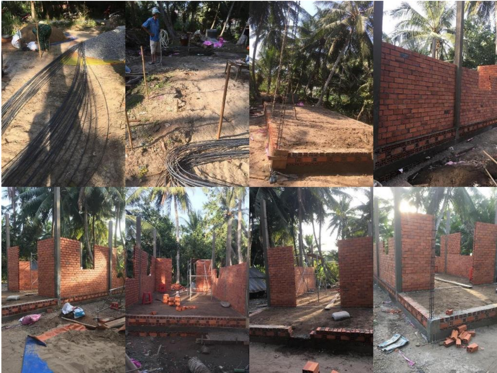
During Construction Đang Khi Xây
