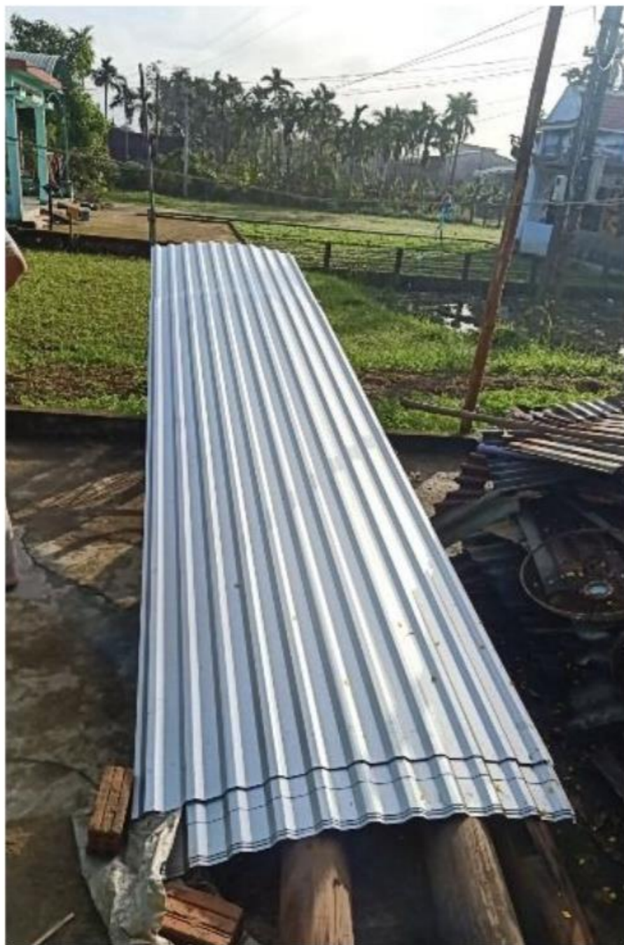
During Construction Đang Khi Xây
